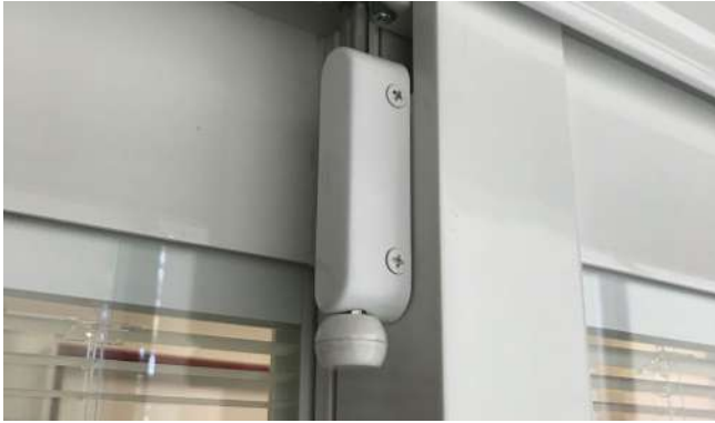
TOP LOCK Optional on Capri door only. The top lock mounts at the top of the operating door and locks into the top of the door frame. With the bolt in locked position, the door cannot operate.
